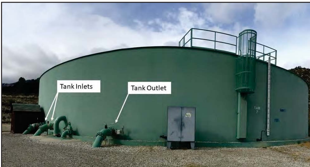
Figure 16: Tank 7 - inlets and outlet
