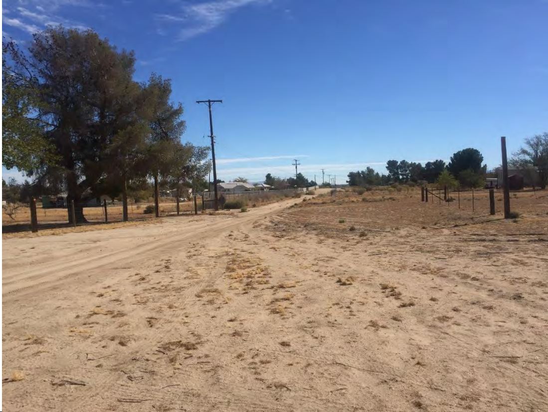
Photo 3. Connecting pipeline alignment; looking east along south side of Walnut Road.
